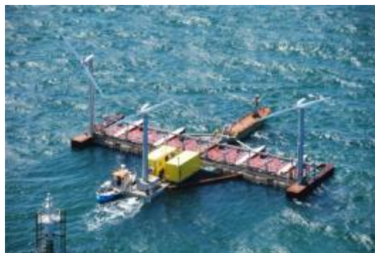
Figure 4: A Floating Power Plant prototype installed off the coast of Denmark
